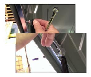
4) Feed one of two supplied M8 x 45mm Hex bolts through the eye at the top of the gas chamber section of the supporting strut. Thread the 2x M8 plain nuts on to the bolt, locking the pair off to leave a small amount of play between the strut and the adjacent fixings.
